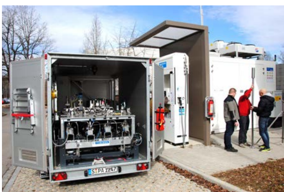
The measuring unit alongside an H 2 filling station. Photo: ZSW
