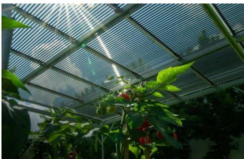
Tubular solar modules from TubeSolar above a tomato field
