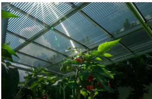
Tubular solar modules from TubeSolar above a tomato field
