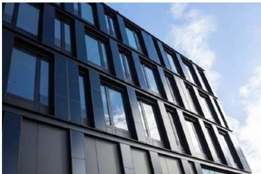
A building-integrated PV system: These CIGS thin-film modules grace the façade of the ZSW headquarters in Stuttgart. Photo: ZSW
