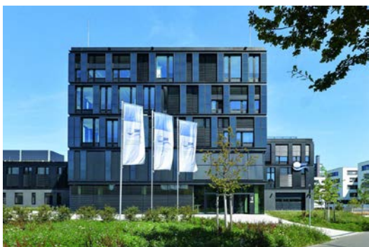
Front view of the ZSW building. Photo: ZSW / www.hochbau-fotografie.de
