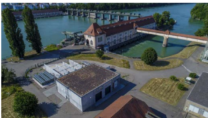
The industrial power-to-gas plant at the Grenzach-Wyhlen hydroelectric power station
