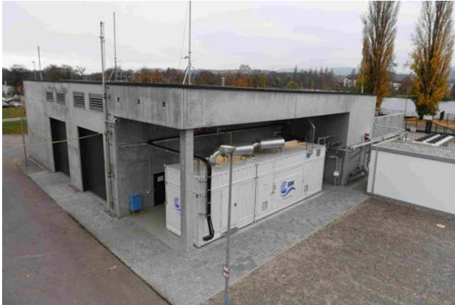
The ZSW's research electrolyser
