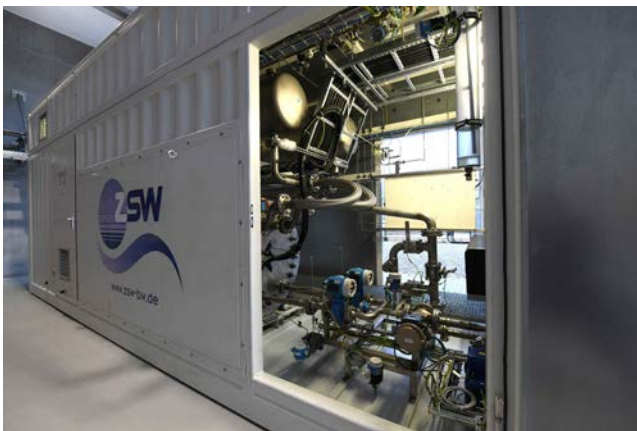
A look inside the plant
