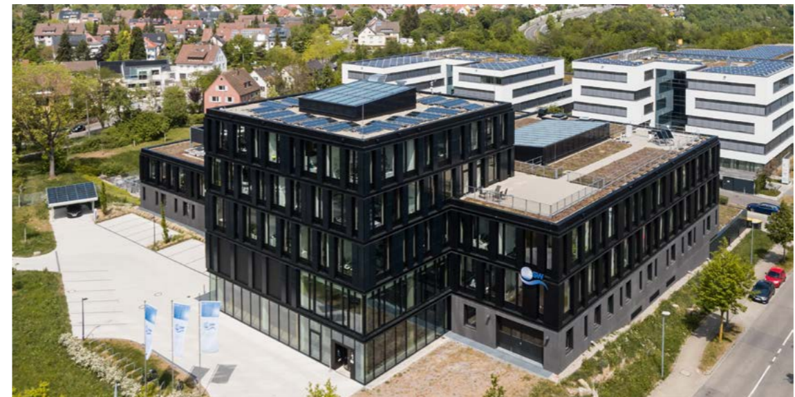
The ZSW buildings in Ulm (top) and Stuttgart (bottom).
