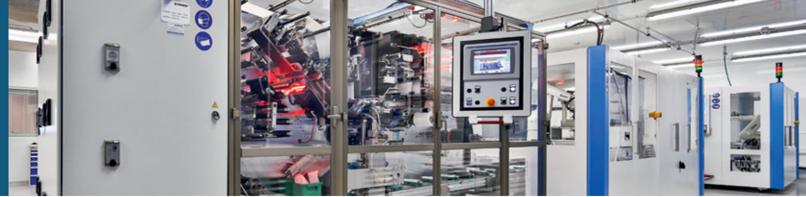
200 m 2 drying room for fully automatic assembly of wound prismatic cells.
