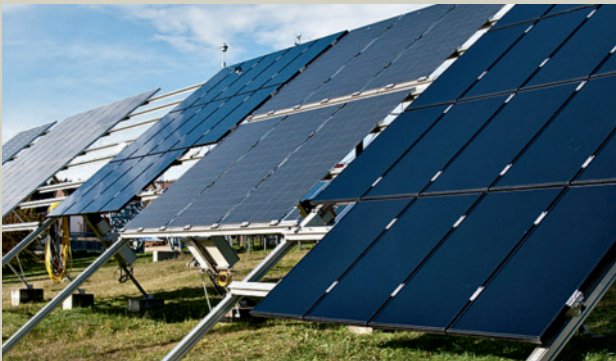
// PV generator test, Widderstall, Southern Germany
