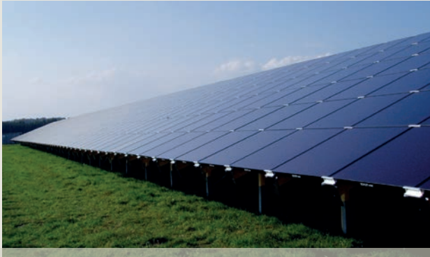
// PV power plant
